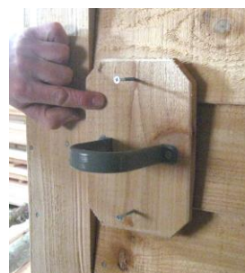
Downpipe support blocks
