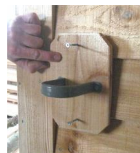
Downpipe support blocks
