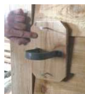
Downpipe support blocks
