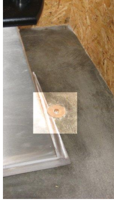
Use pedestal fix down (B4) at rear.
