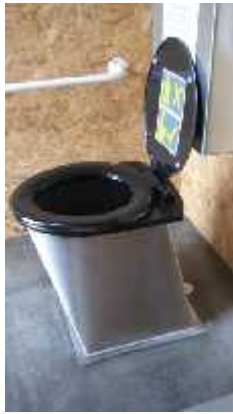
Use pedestal fix down (B4) at rear.
