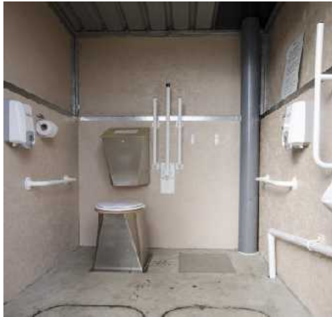
Metal building interior
