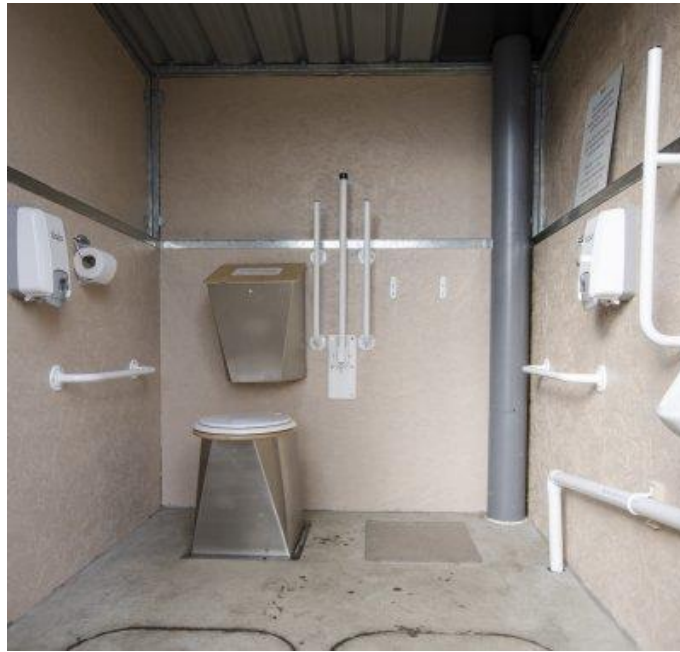
Metal building interior
