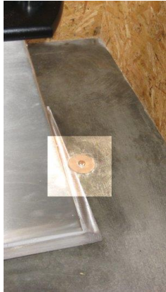
Use pedestal fix down (B4) at rear.
