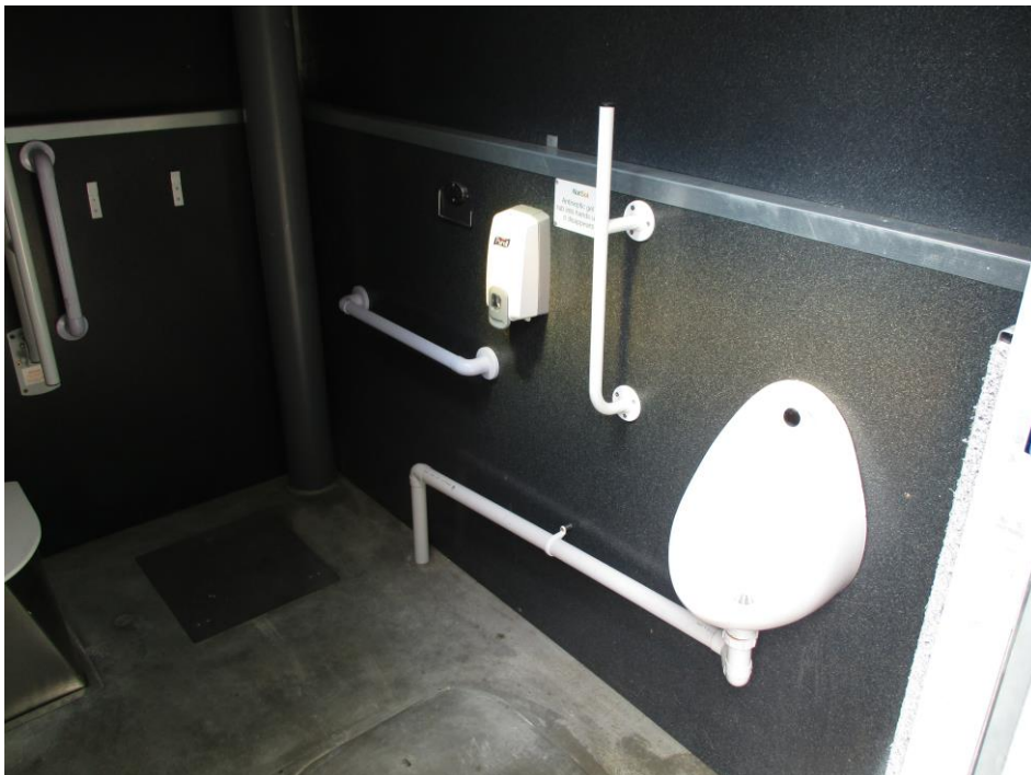
Urinal fitting and grab rails.
