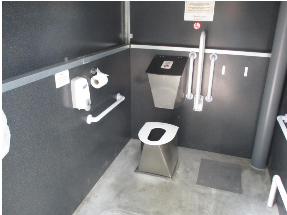
Metal building interior – walls are lined with EkoPly recycled plastic board. They should have been marked with black felt tip to show the positions of fittings.
