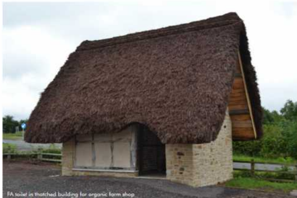
FA toilet in thatched building for organic farm shop
