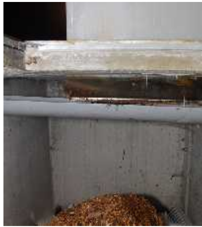
Checking urine gutter
