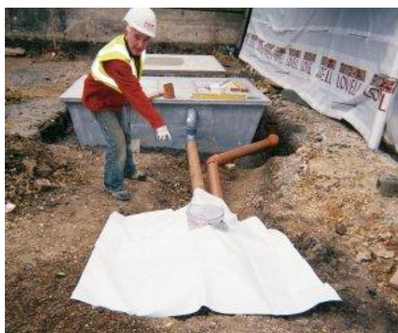
With rainwater – use separate pipe
