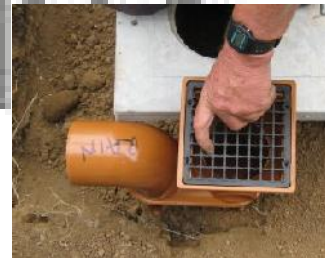
Possible rain gully position
