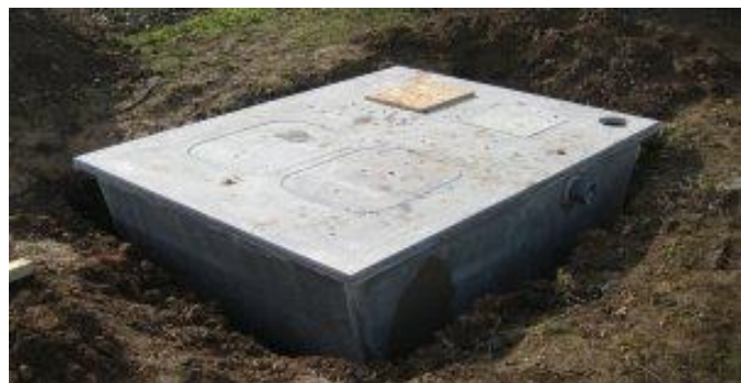
A view from the front RH corner of the building. The ventilation socket is in the back RH corner.
