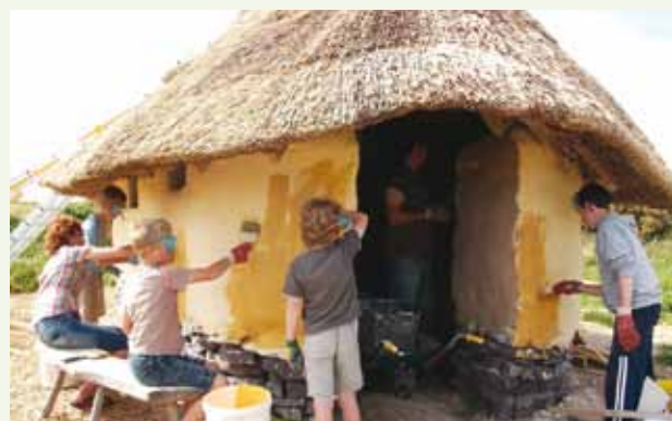
Young volunteers helping to limewash the walls of the toilet
