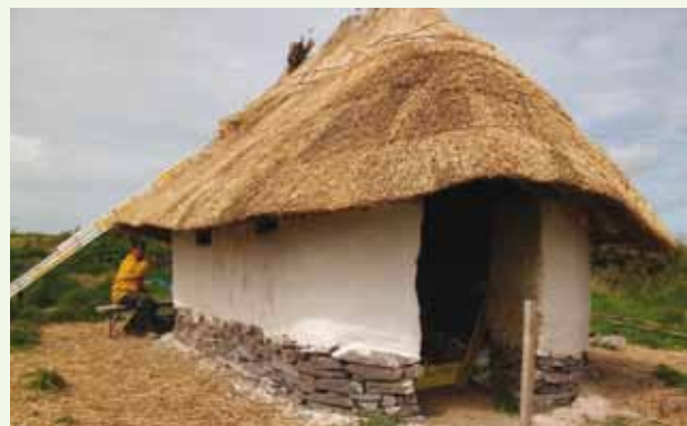
Limewashing the compost toilet
