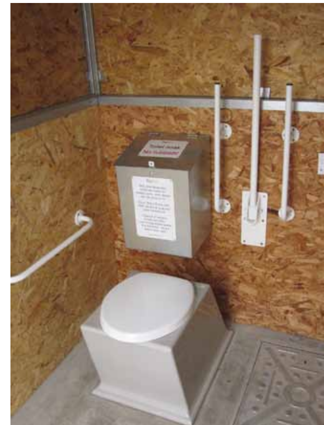
The interior of a compost toilet built on the Forest Farm Allotments in Wales.
