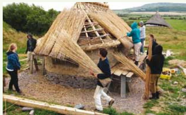
Putting thatch on the compost toilet roof
